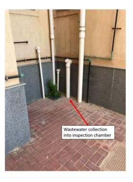
Collection of wastewaters (separate pipes of grey and black water) from each flat Wastewater collection into the inspection chamber, and then transferred by underground drainage pipes into the public sewer system
